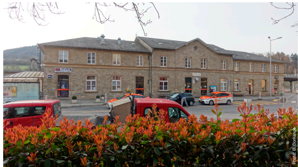
Figure 5. View of the Ettelbruck train station.
