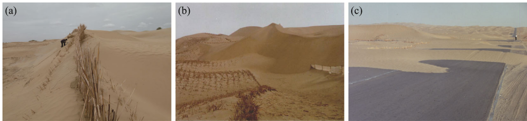
Fig. 2 Damage conditions of the mechanical sand control system caused by wind-blown sand along the Taklimakan Desert Highway. (a), buried sand barrier fences; (b), sand aggregation in the straw checkerboard barriers; (c), moving dune coverage on the desert highway.
