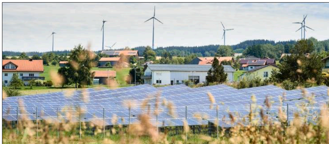
Fig. 14. Wind turbines and solar panels at Wildpoldsried [113].
