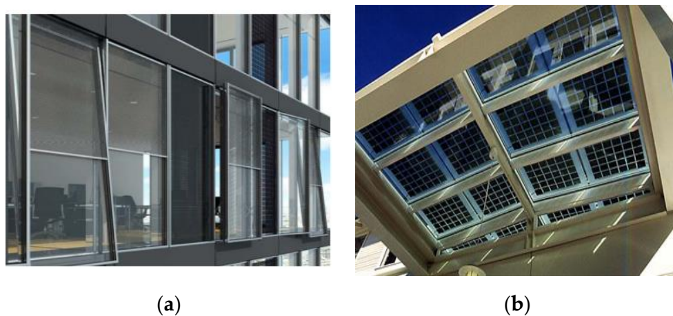
Figure 9. (a) BIPV façades powered by electricity to assist natural ventilation [186]; (b) an entrance with a PV skylight [187].
