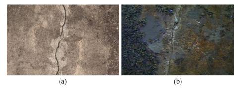
Figure 6. Crack image: (a) crack image taken in the air; (b) crack image taken underwater.
