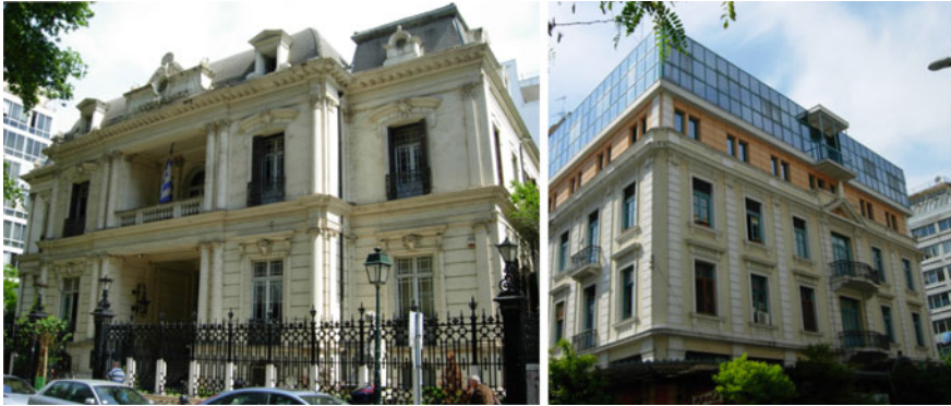
Fig. 1 Heritage buildings of the 20th century located at the center of Thessaloniki, Greece
