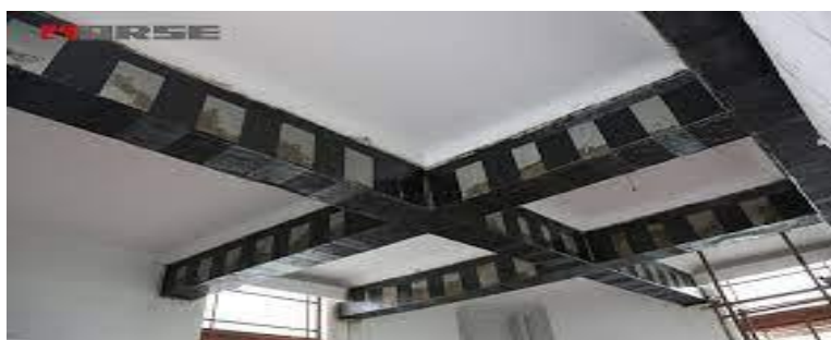
Figure 5. CFRPs in beams
