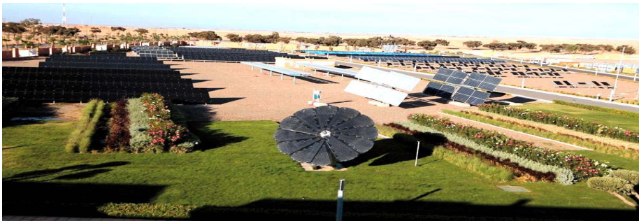
Fig. 5. Photo of the Solar Test Facility, 100 kW p different PV technologies installed at the Green energy Park (GEP), Benguerir, Morocco
