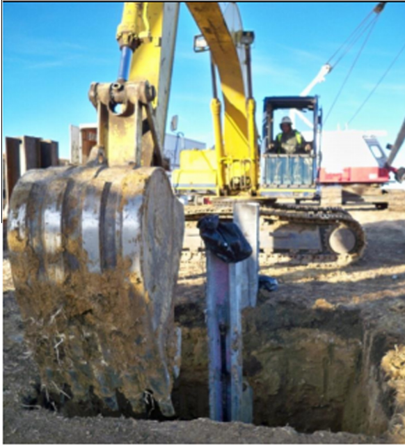
Fig. 17. Excavation of soil surrounding P4.
