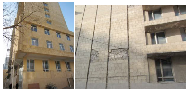
Fig.3. Photographs of second educational building of AzUAC
