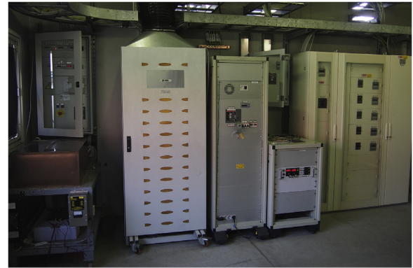
Fig. 6. Photo of the RSE dc microgrid.
