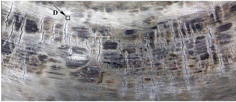
Fig. 3. Closeup view of the local friction surface.
