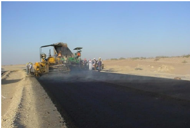
Figure 4. Fumes released from behind the paver
