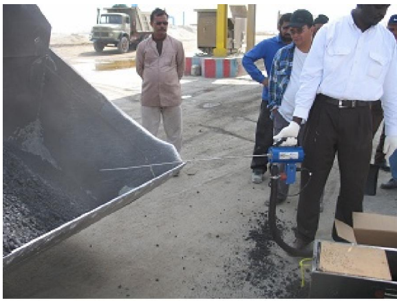
Figure 2. Air quality monitoring at the asphalt plant
