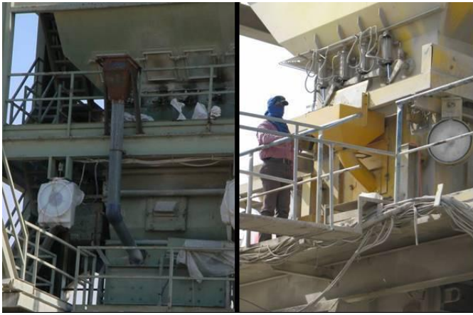
Figure 1. Local modified asphalt batch plants
