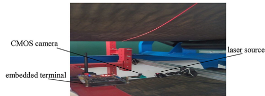
Fig. 12. The monitoring system.
