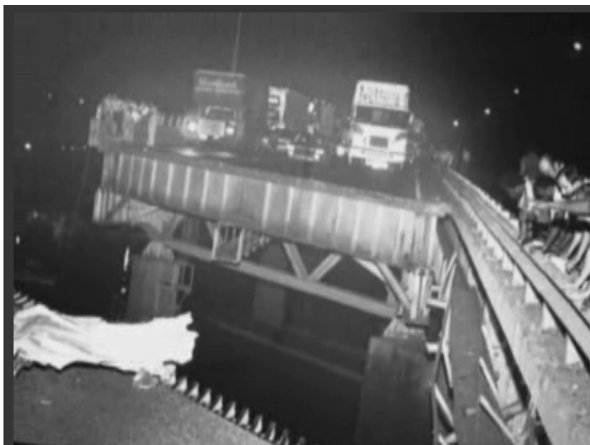
Mianus River Bridge Collapse – June 28, 1983
