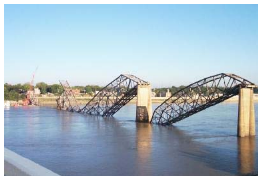
Cape Girardeau Truss Demolition
