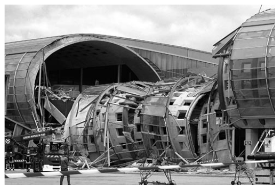
Fig. 15 Partial collapse of the Charles de Gaulle Airport Terminal, Paris
