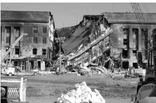
Fig. 14 Partial collapse of the Pentagon Building
