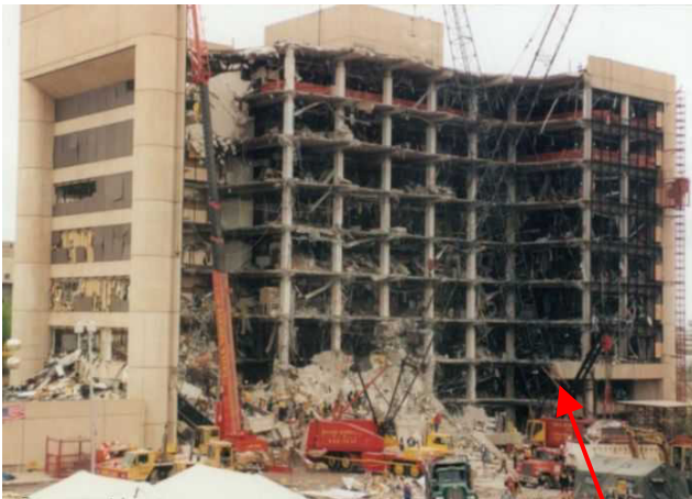
collapse stopped at rebar discontinuity in transfer girder
