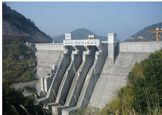
(a) Downstream view of the dam
