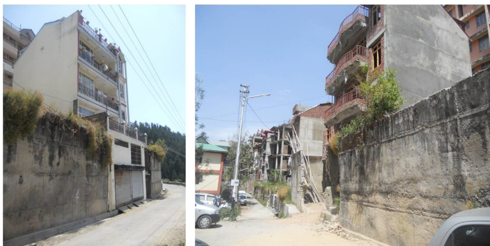
Fig. 15. Addition of extra storey after demolition of retaining walls in New Shimla.
