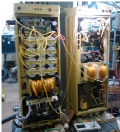
Figure 10. Frequency converter (boost converter is on the left)
