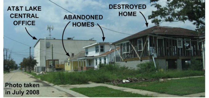
Fig. 13. AT&T's Lake CO in New Orleans and its surroundings.
