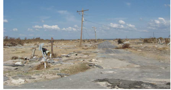
Fig. 9. Gilchrist, TX, after Hurricane Ike.
