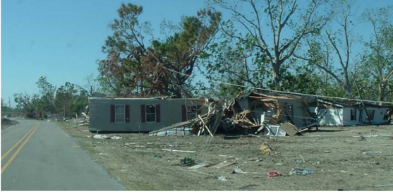
Fig. 11. Near Point a La Hache, LA, after Hurricane Katrina.
