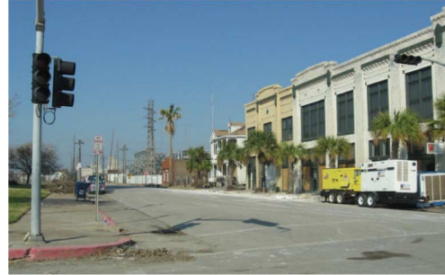
Fig. 10. Galveston, TX, after Hurricane Ike.
