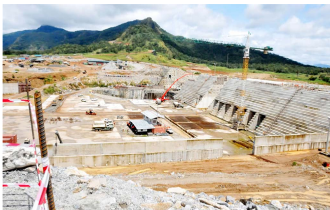
Fig. 10. Mambila hydro power plant sites under construction [63].
