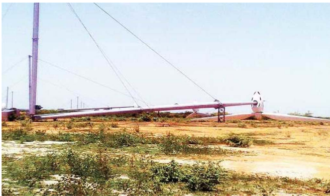
Fig. 12. 10 MW wind farm site at Rimi, Katsina State [73].
