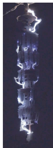
Figure 11. Flashover path of composite insulators
