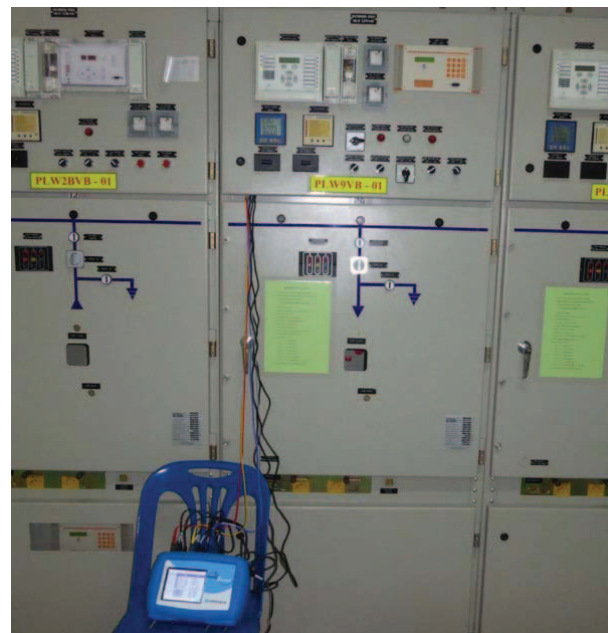
Fig.7 Power quality measurement set up at the Plauk Deng 3 substation
