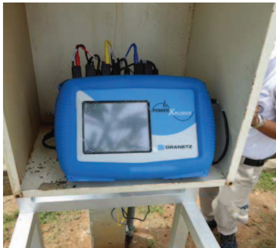
Fig.9 Power quality measurement set up at the PCC (Solar PV rooftop station)
