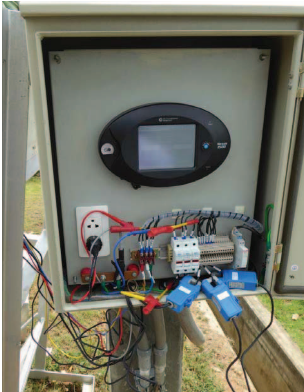
Fig.8 Power quality measurement set up at the PCC (Solar PV rooftop station)
