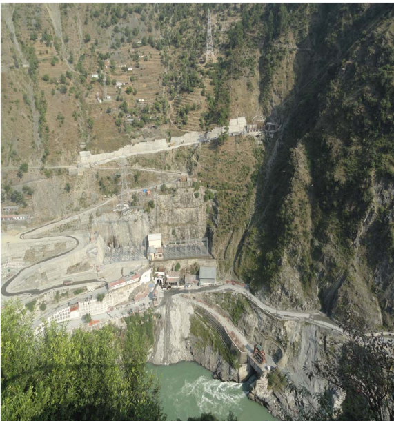
Fig. 7. Power house of Baglihar hydro power project constructed on the Chenab river in J & K. Source: Author's own contribution.
