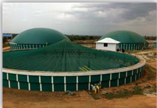
Fig. 6. Bio-methanation plant in Tamilnadu.
