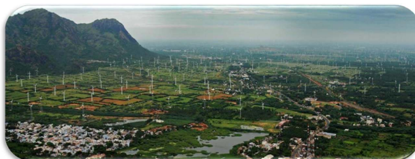
Fig. 5. Muppandal wind farm in Tamilnadu with 1500 MW of installed capacity.
