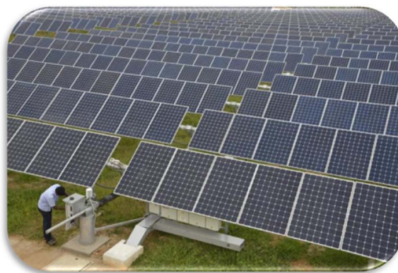
Fig. 8. Grid connected 1 MW solar power plant in Tamilnadu under REC scheme.
